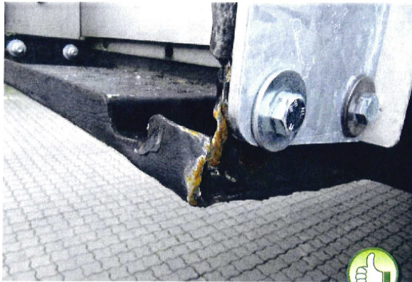
Lead in plate Correctly executed repair
